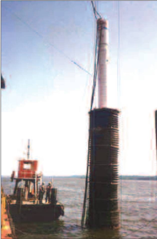
Figure 3.11 The IHC S-280 hammer in use.
